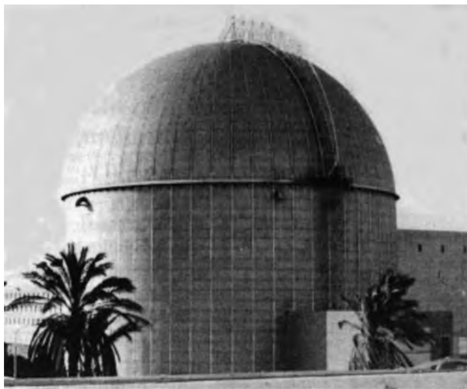
The Dimona Reactor Dome Credit: Mordechai Vanunu
