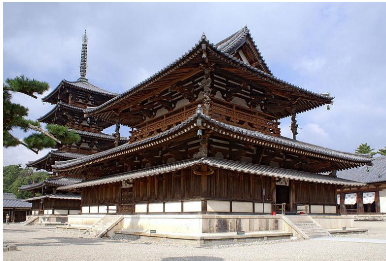
The Golden Hall and five-storey pagoda of Hōryū-ji, among the oldest wooden buildings in the world, National Treasures, and a UNESCO World Heritage Site
